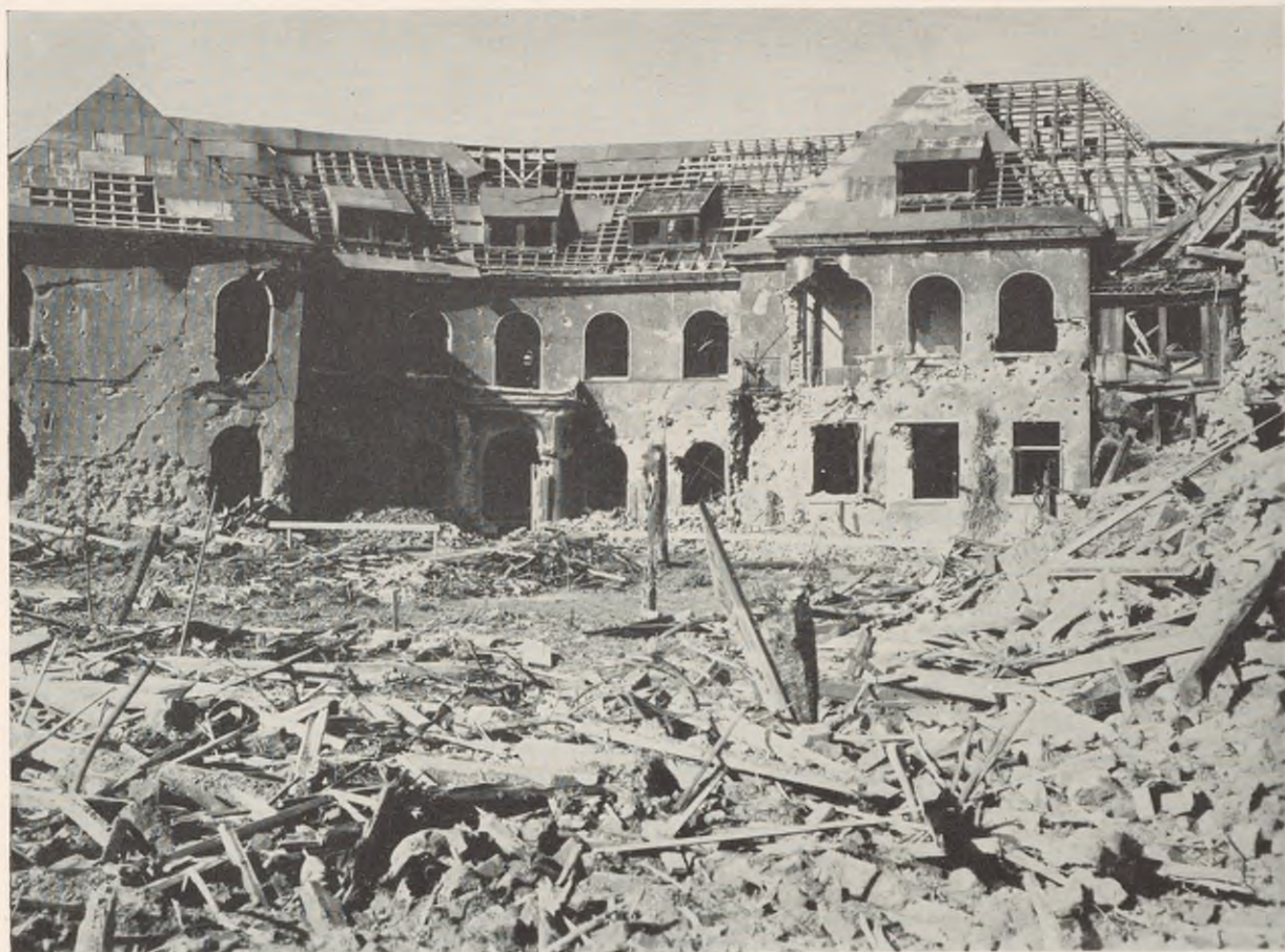
FIGURE 108. Obstetrics and gynecology clinic of the Krupp sanatorium which was taken over when main hospital was destroyed (Fig. 72). Land mine hit just this side of building doing all damage shown. Two nurses were killed. Building is regarded as "moderately damaged."
