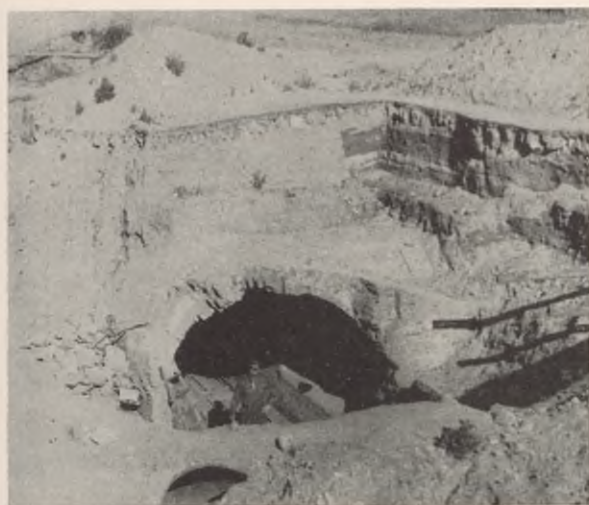
FIGURE 141. Trunk sewer blown open by direct hit during air raid. Damaged water main at left.
