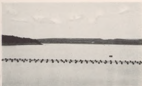
FIGURE 138. Moehne Dam. Nets installed after reconstruction to prevent floating mines from hitting dam.
