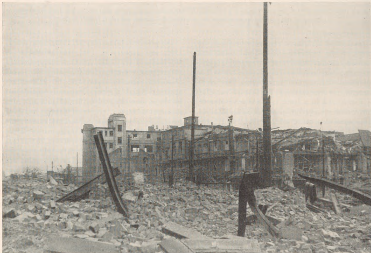
FIGURE 167. Knoll plant viewed from grade crossing on western boundary of plant property. Power plant is to extreme right, center is chemical synthesis building. The granulating department and the towered building for filling, packaging and storage of finished supplies is shown in the background. All buildings are severely damaged or completely destroyed, i.e., will have to be taken down to their foundations and entirely replaced.
