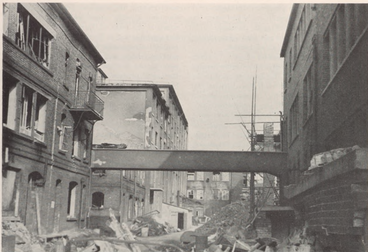
FIGURE 170. View of destruction inside plant area. Granulating and coating building is to the left while rear of administration building is to the right. Most of damage visible here is from blast effect only.
