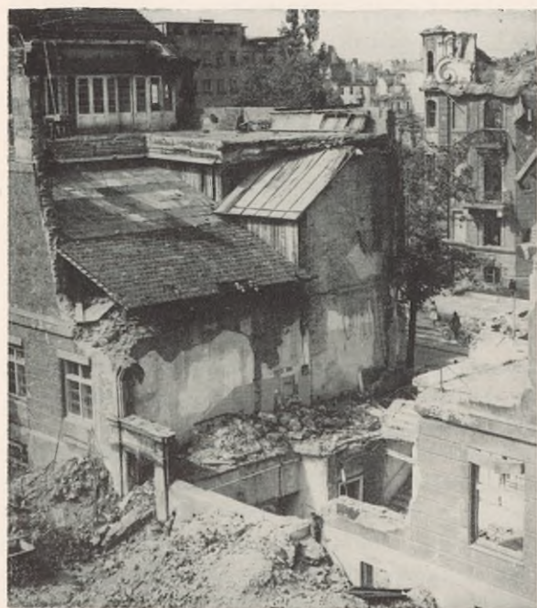
FIGURE 61. Air raid damage to Eye Clinic, University of Munich.
