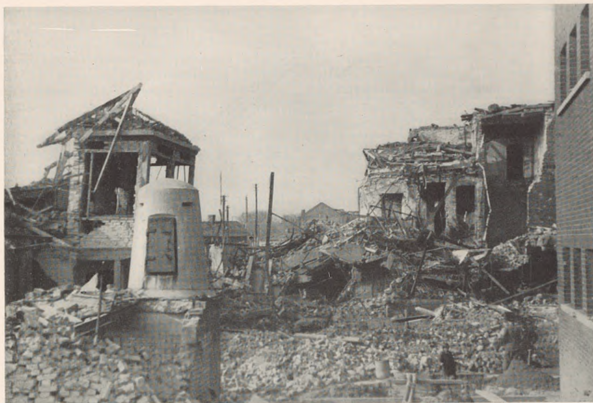
FIGURE 169. Looking north from main entrance to the plant showing total destruction of chemical synthesis, boiler and turbine buildings (buildings 3, 5, and 6 in Figure 169). Warden in look-out post (left foreground) was unhurt.
