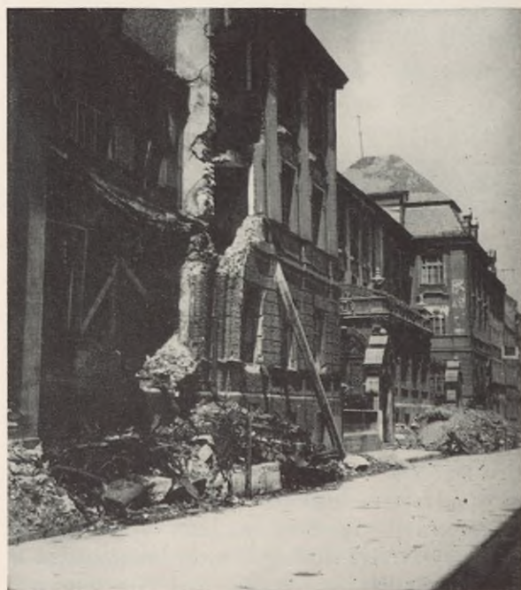
FIGURE 60. Air raid damage to Children's Clinic, University of Munich.
