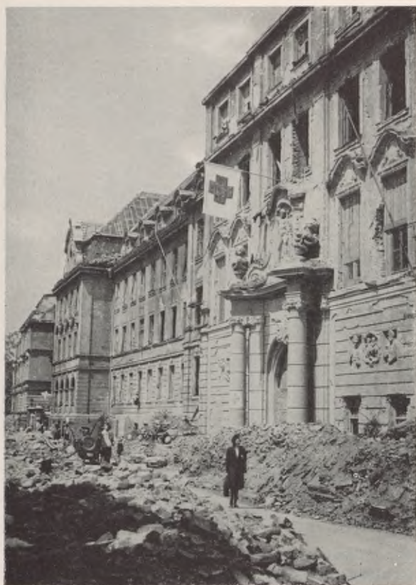
FIGURE 62. Air raid damage to Polyclinic Building, University of Munich.
