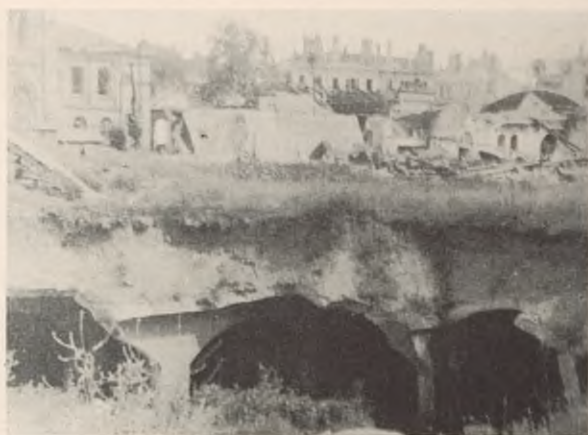
FIGURE 125. Bomb damage to 2.5 million gallon reservoir—Cologne.
