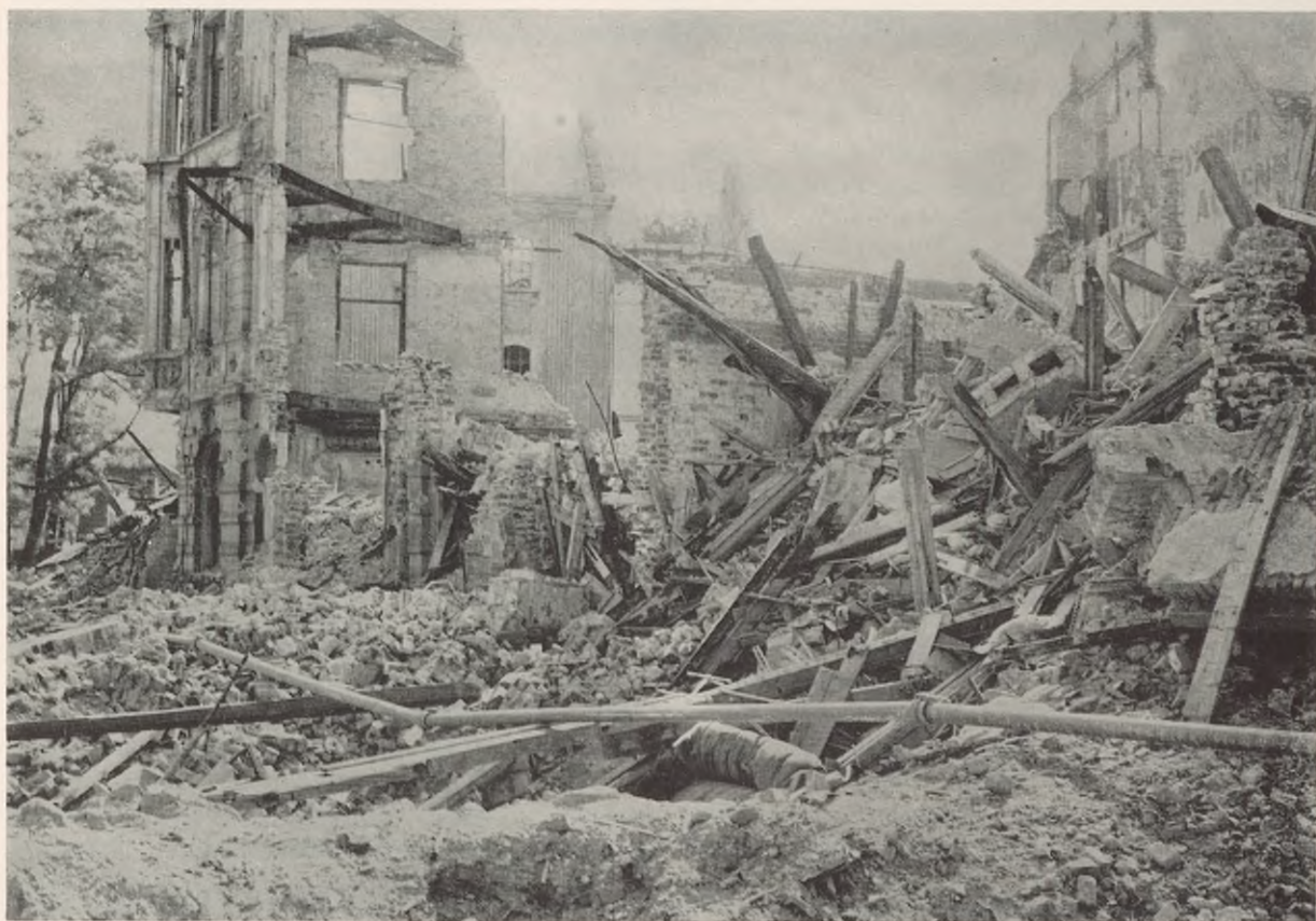
FIGURE 132. Emergency water line. Hastily laid across rubble following an air raid.
