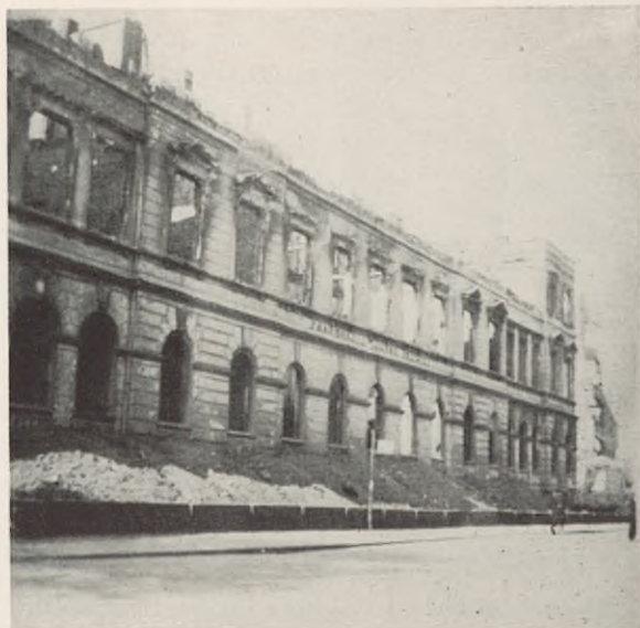
FIGURE 67. Damage to Pharmacology Building, University of Leipzig, by air raid of 4 December, 1943.
