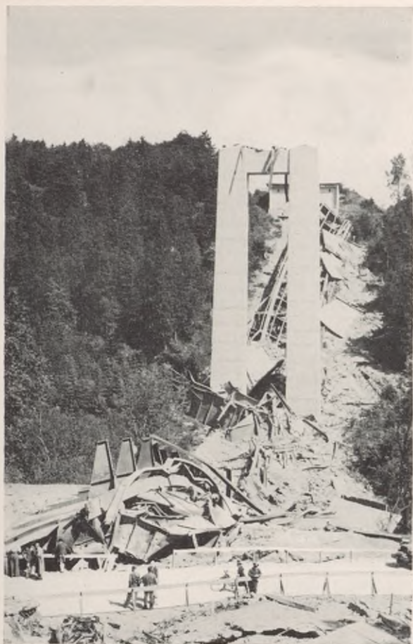
FIGURE 123. "Scorched earth" destruction to transportation and water supply lines. Remains of Reichsautobahn (Highway) bridge over Mangfall river destroyed by the Germans after American troops had crossed. Broken water supply line to Munich lies under steel wreckage in foreground.
