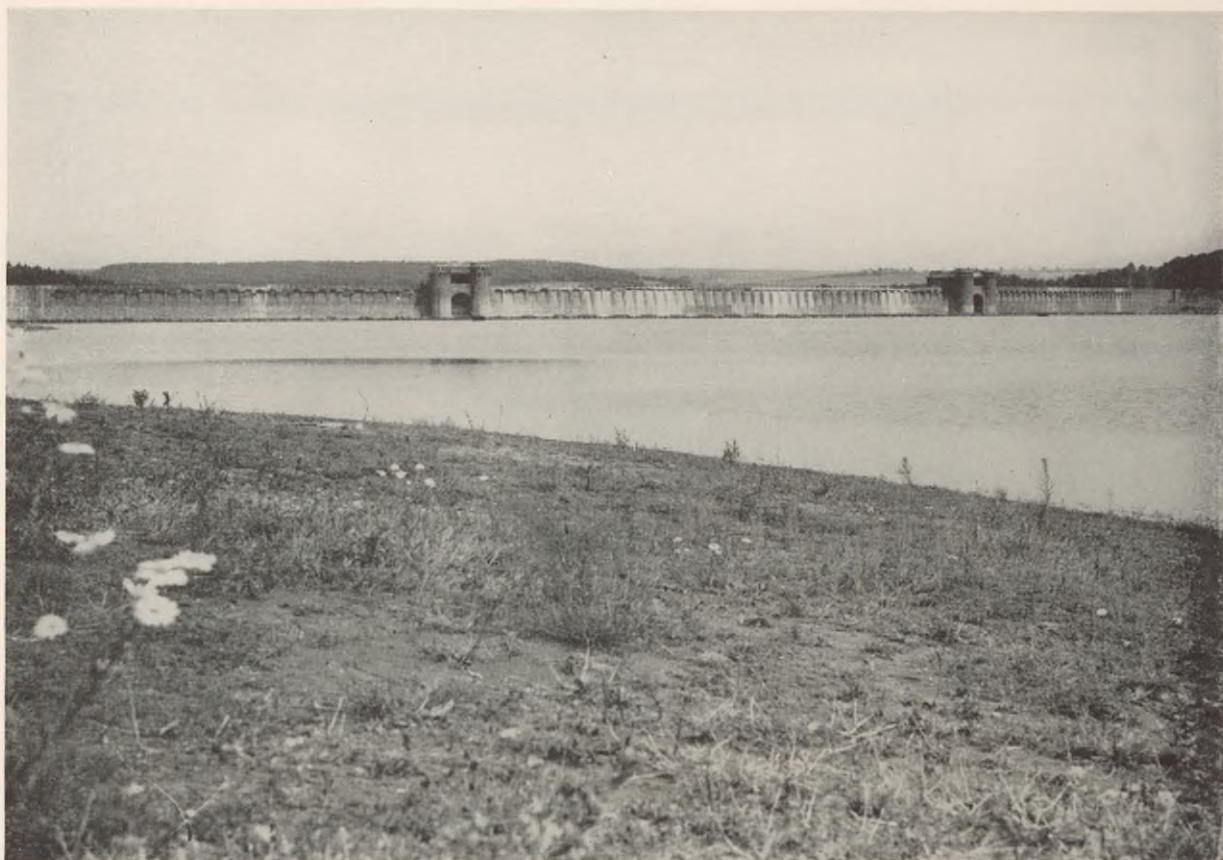
FIGURE 136. Mochne Dam, upstream side, after reconstruction. Water level maintained at halfway mark to reduce flood damage should dam be rededstroyed.
