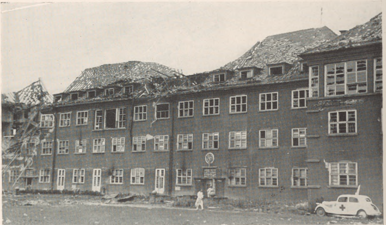
FIGURE 102. Internal medicine clinic at Ludwigshafen municipal hospital. First two stories were still in use despite the damage.
