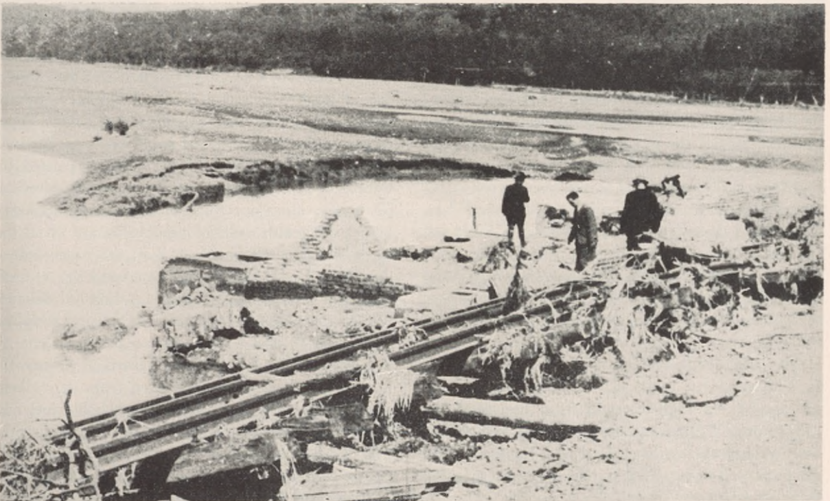
FIGURE 134. Remains of water works at Neheim. Destroyed by the flood when the Moehne dam was destroyed by direct aerial bombardment—May, 1943.
