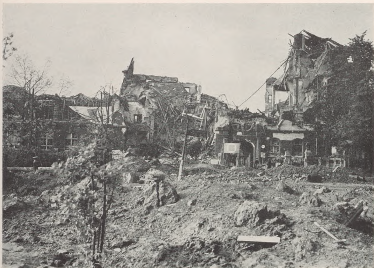
FIGURE 109. Municipal hospital, Essen, showing what was left of administration building and out-patient clinic. Half of this structure was functioning when visited. 116 high explosive bombs fell within the grounds of the hospital, of which this hospital is a part, during a single raid. Bed capacity was reduced from 700 to 120.
