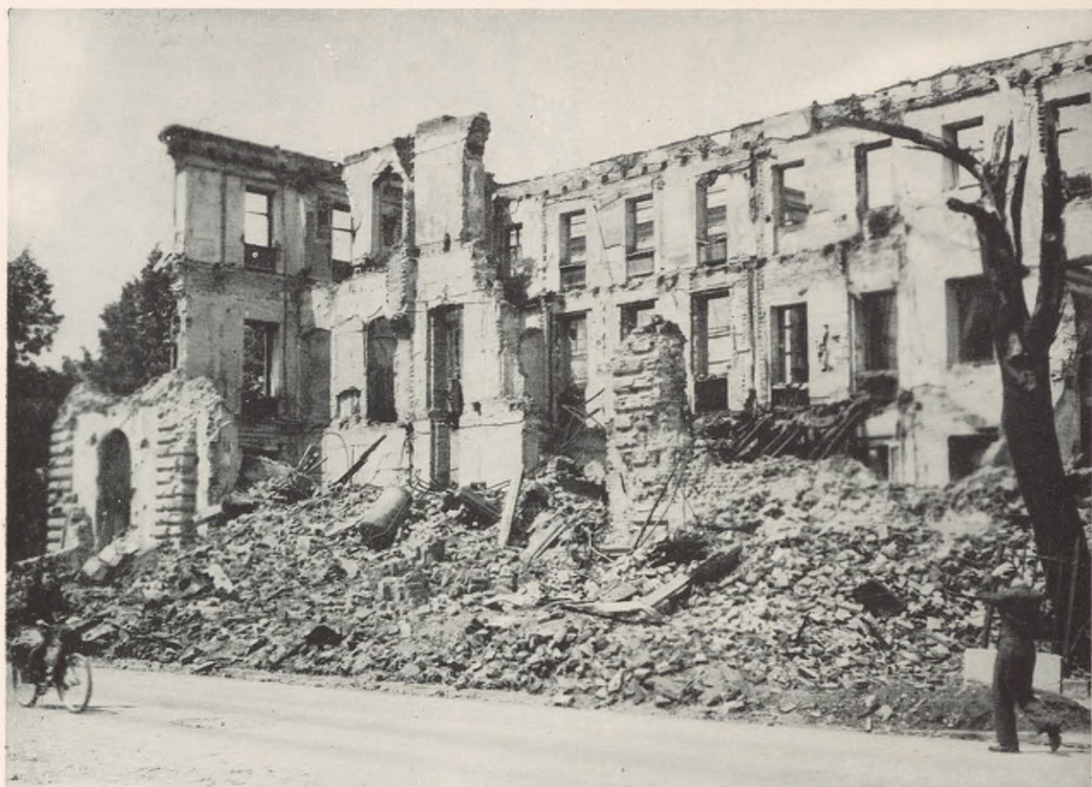
FIGURE 59. Air raid damage to Second Medical Clinic, University of Munich.
