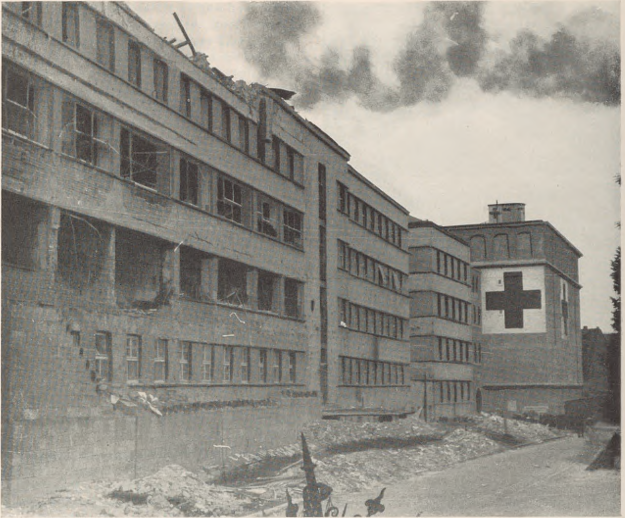
FIGURE 90. Bunker hospital at Nuremberg showing connection to main building. The obstetrics and gynecology clinic on the left had been damaged by a bomb hitting in the courtyard on the other side of the building. Appendage atop the five story windowless hospital is a fire watcher's shelter. Walls, roof and floors are nine feet thick.
