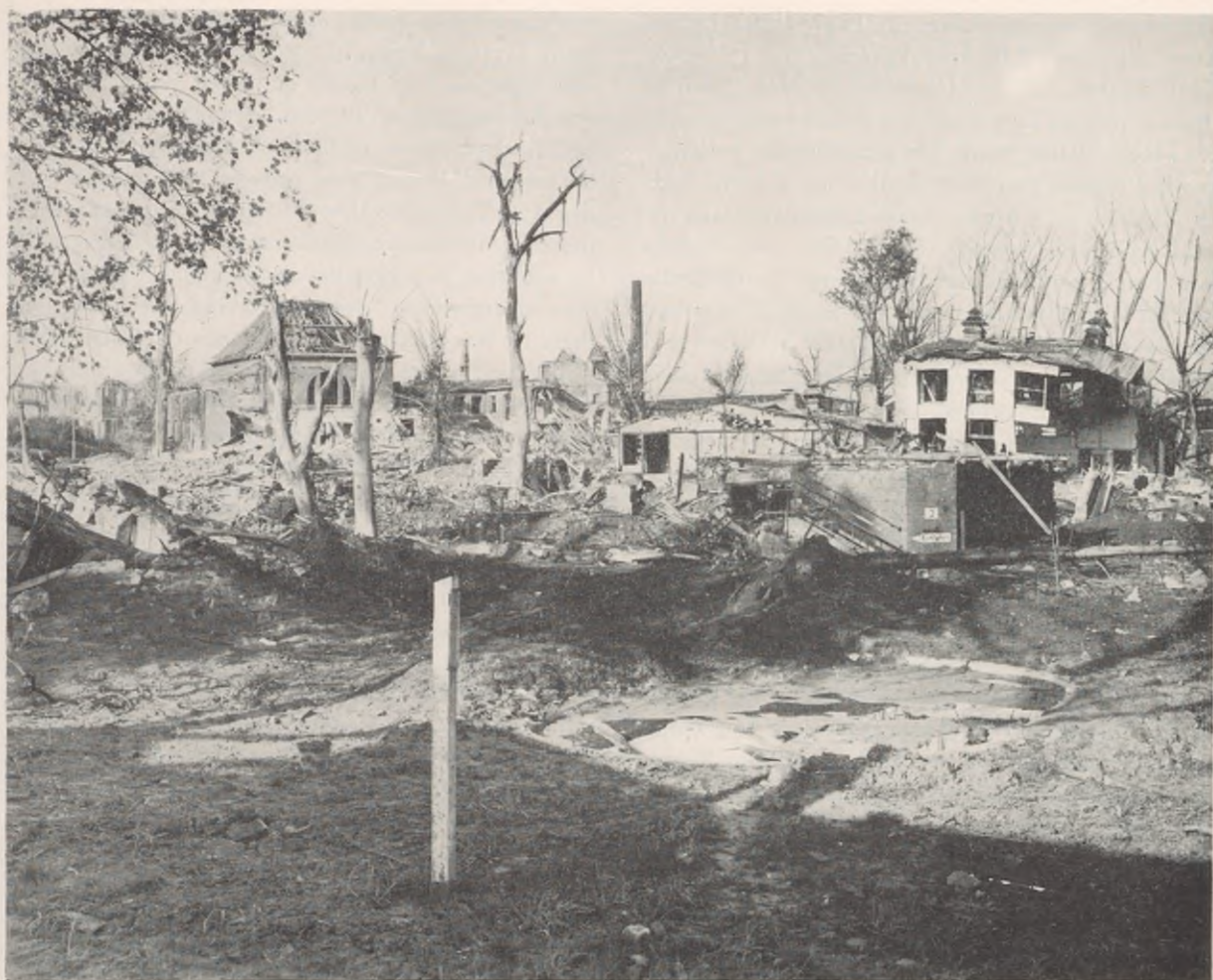
FIGURE 72. Air raid damage to Krupp Hospital, Essen. This was one of the most modern installations in Europe and was completely destroyed in one raid. Hospital grounds were adjacent to main Krupp Works.
