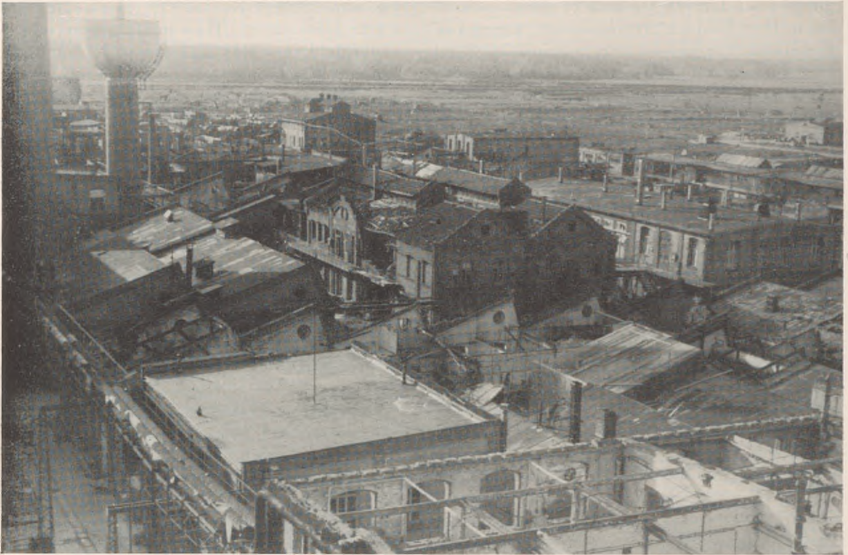
FIGURE 193. Merck plant view of damage to buildings for manufacture of inorganic salts (foreground) and for reagents and rare chemicals (to right of tower). Buildings are numbers 11 and 12 in chart on Figure 194.
