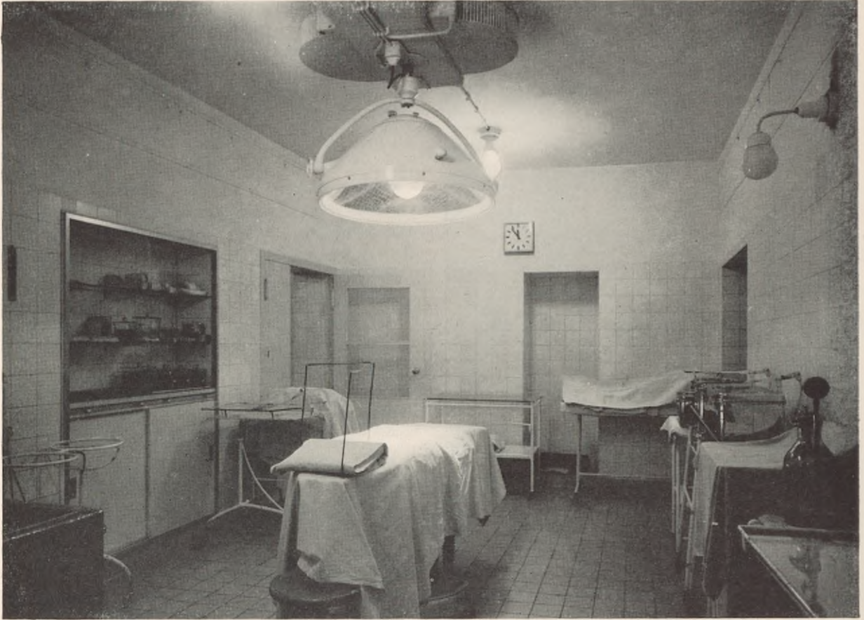
FIGURE 99. Air raid hospital bunker, Frankfurt on Main. Operating room. The operating rooms were connected by the hallway shown through the doorway in rear. This hallway provided access from all rooms, to the central sterilizing room. There was one scrub room for each operating room.
